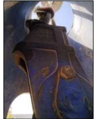
Crane wedge sockets & Wire Ropes Termination found satisfactory at the time of inspection
